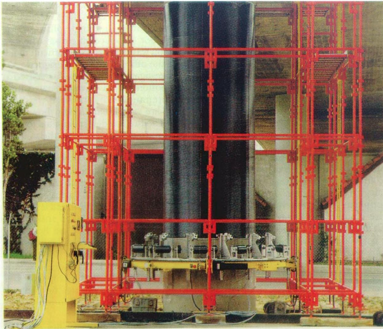
**JACKET** Computer-controlled robot wraps concrete columns with carbon fiber.
