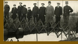
Folding bridge for emergencies: The emergency bridge can easily be transported as a suitcase. Invented by G. Durré. The Netherlands, 1976.
