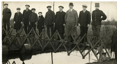
Folding bridge for emergencies: The emergency bridge can easily be transported on a handcart; invented by L. Deth. The Netherlands. 1926
