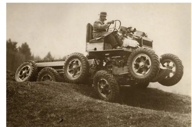
All-terrain car: This all-terrain car can descend slopes up to 65 degrees; England, 1936.
