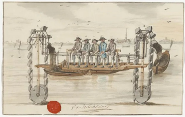
Manual dredger: Workers operated the so-called bucket dredger with their arms and legs using stepper boards.
