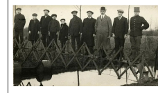
Folding bridge for emergencies: The emergency bridge can easily be transported on a handcart; invented by L. Dech. The Netherlands, 1926.
