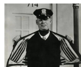
Electrically heated jacket: developed for the traffic police in the United States, 1932. The power is supplied by electric contacts in the street.
